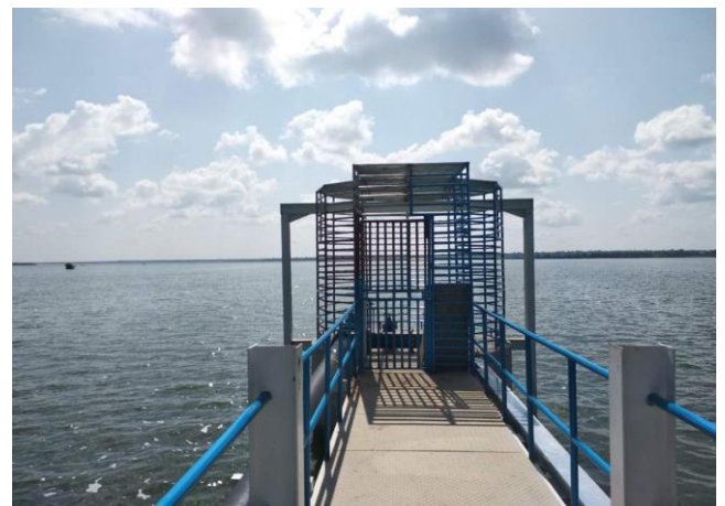
Picture 4.2: Completed structure with security cage installed
