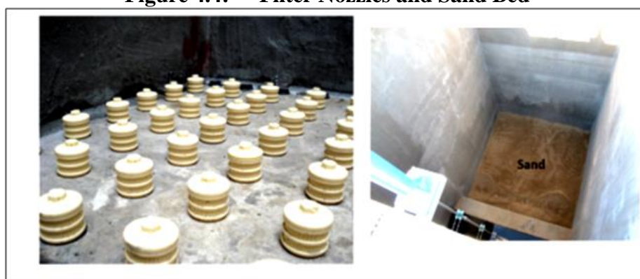
Figure 4.4: Filter Nozzles and Sand Bed
