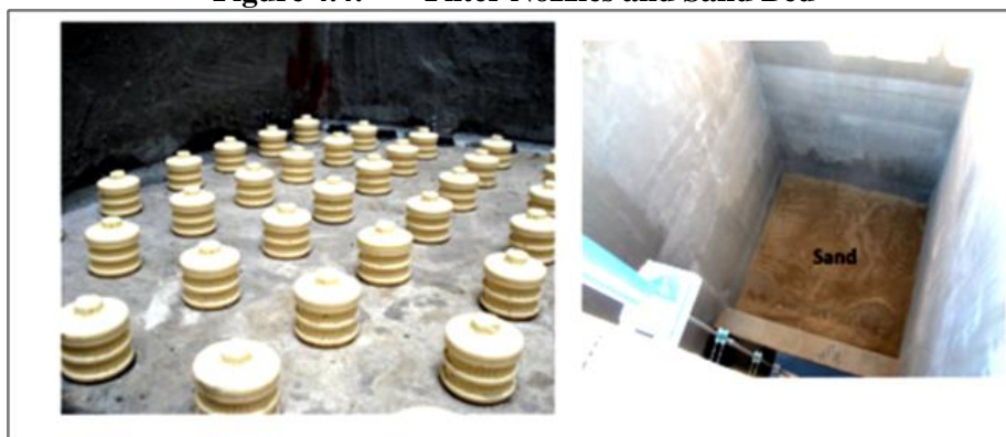
Figure 4.4: Filter Nozzles and Sand Bed
