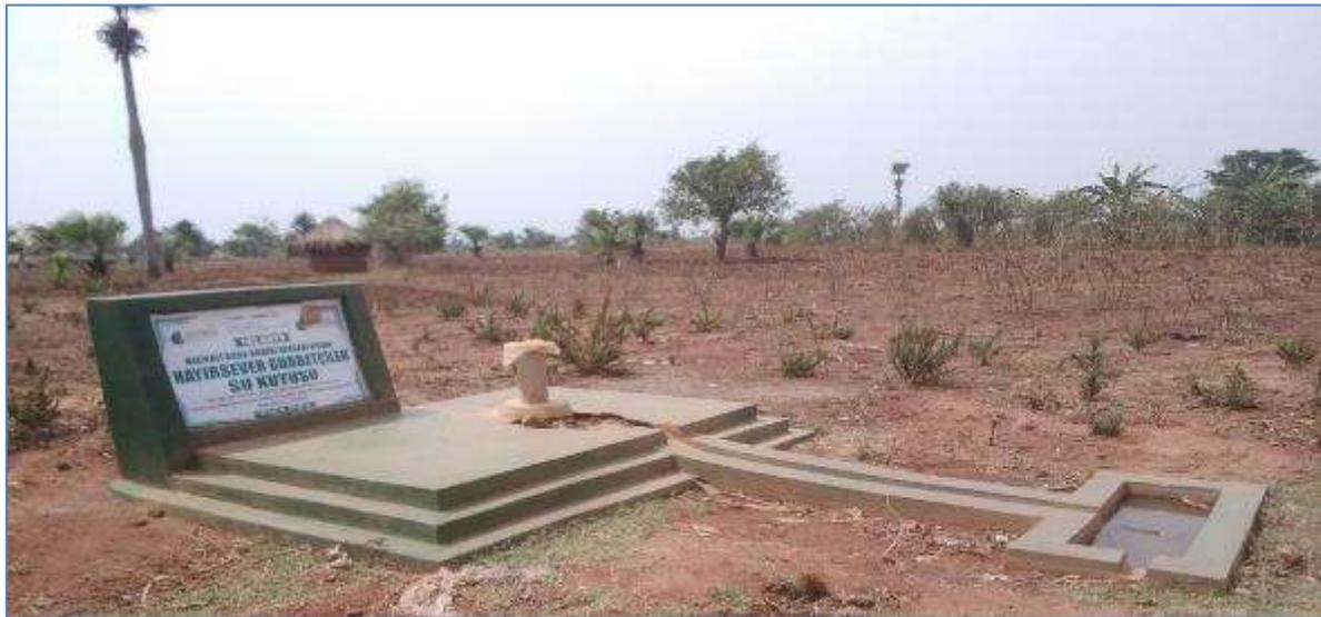
Figure 6-54: Non-functioning deep borehole at Bumogoli village
