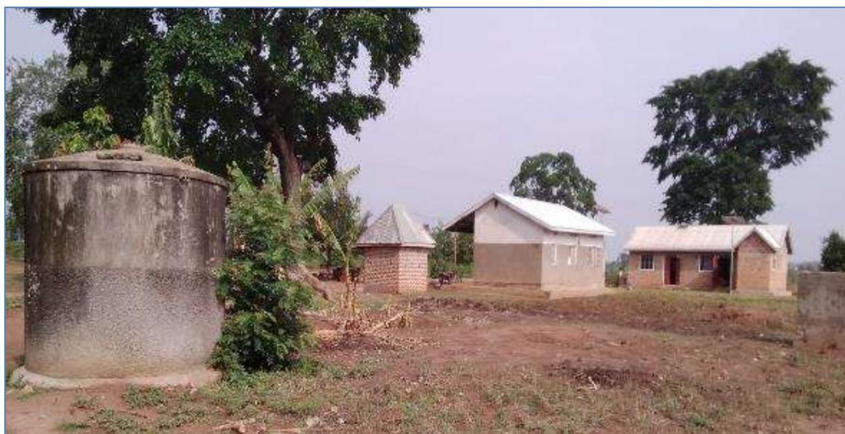
**Figure 6-64: Damaged concrete water tank at Kagulu HC III**
