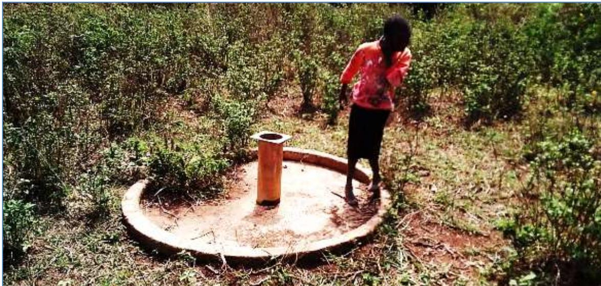
Figure 6-55: Abandoned deep borehole at Nabuuku village in Igwaya RGC
