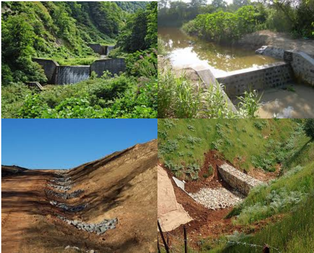
Figure 5 - Sample of Check Dams
