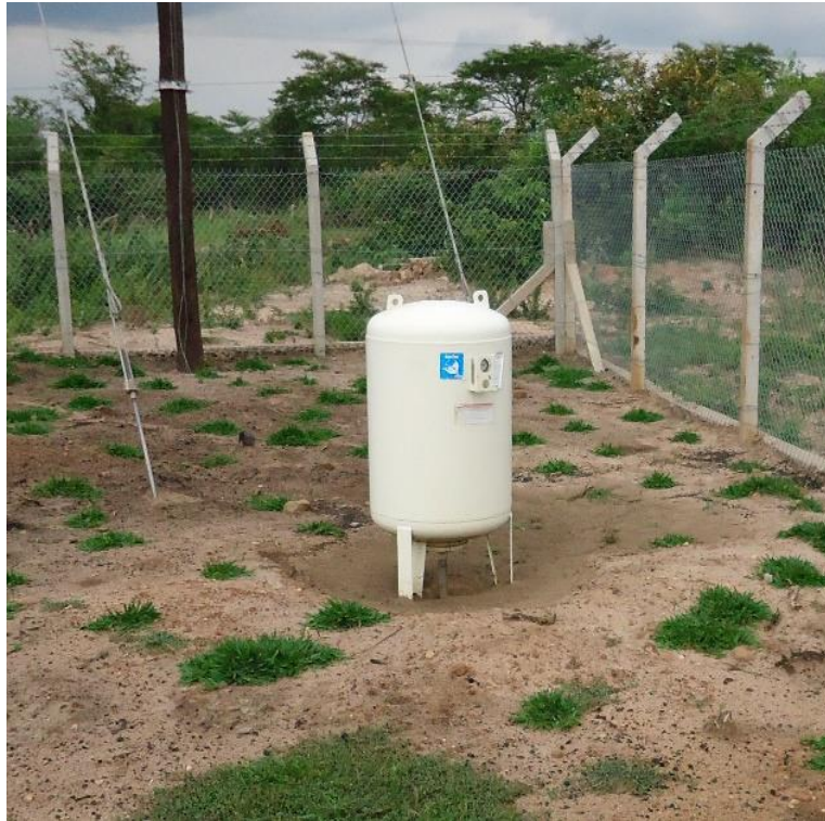
L: Surging controller in Nyamarunda WSS; R: An aerobic digester at NWWTP , Bugolobi Kampala
