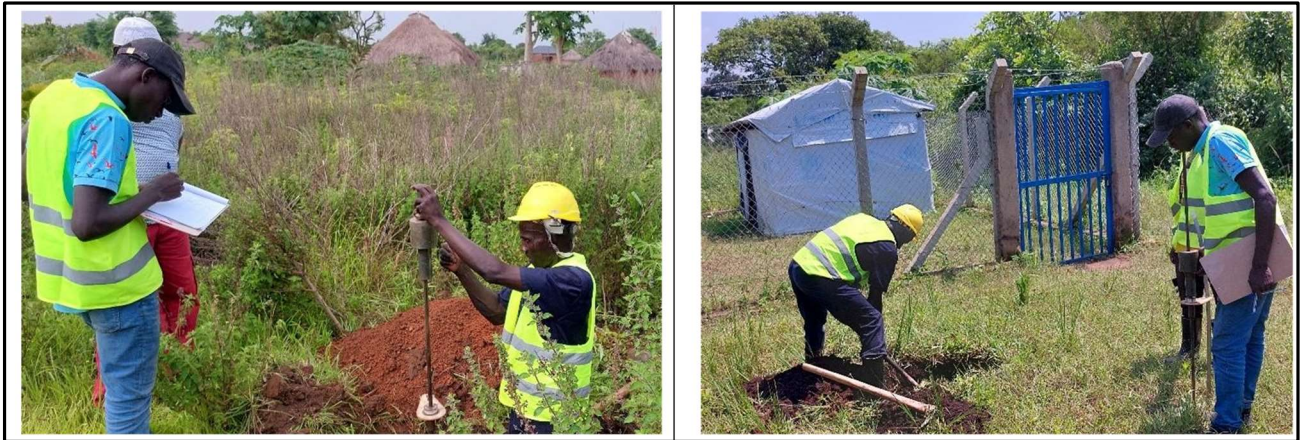
Plate 2-2: Field Activities for Geo-technical Site Investigations (Kaaga and Partners 2023)
