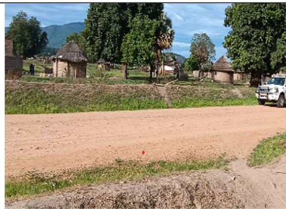
Figure 6-18: Gravel Road within Laropi GRC
