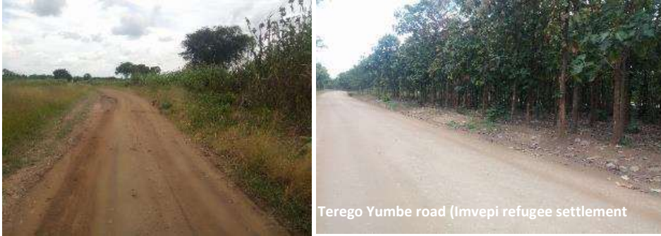
Plate 8.1: Some of the project area roads whose road reserves will host the proposed project
