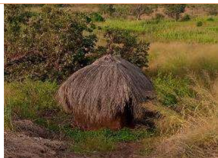
Plate 5.11: A typical sanitary facility in Andiku village
