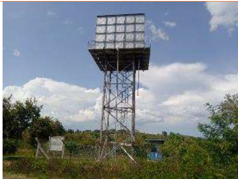
Plate 5.7: Imvepi Safe Water Project in Imvepi Settlement Zone 2 provided by UNICEF and Water Mission Uganda
