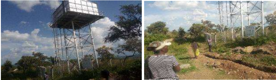
Figure 1-6 : Existing tank at Invepi Refugee Settlement in Nyaranga Village
