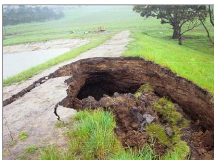
Failure of the wall of a small dam
