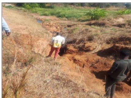
Extensive erosion of the downstream embankment and foot-slopes of a small dam
