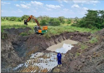
Construction of an excavated valley tank in hydromorphic grasslands in flat terrain
