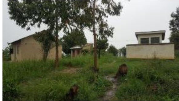
Figure: One of the toilet facilities within the model village
