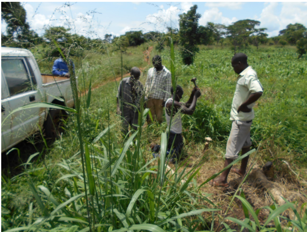
Marking site using a wooden peg
