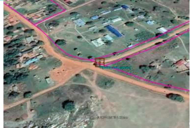
Google image of the Kabugudho Road crossing
