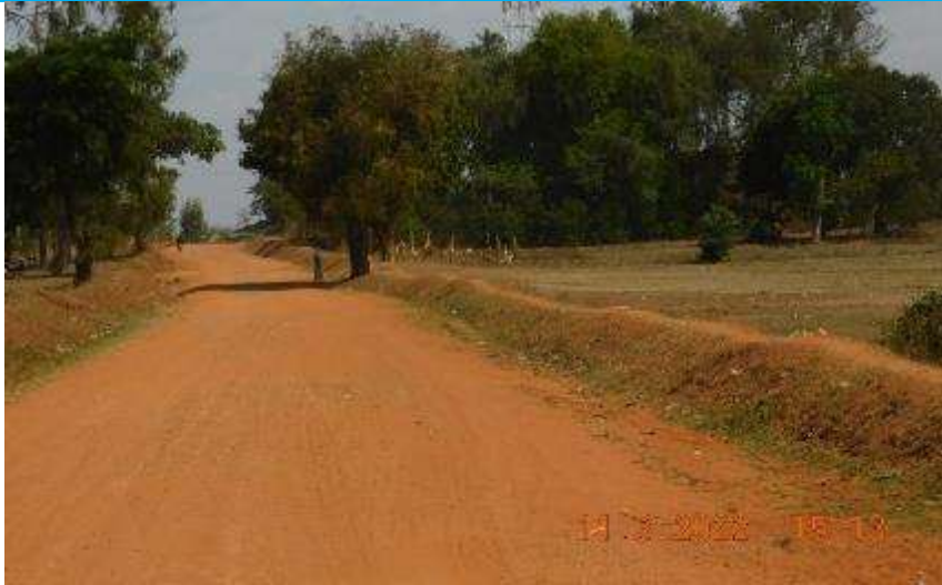
Kabugudho Road crossing
