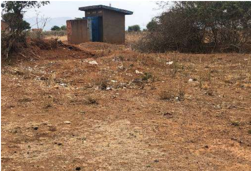
Figure 5-19: Sanitation facilities in the GRC.
