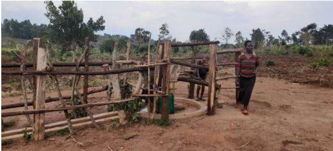
Plate 12: One of the hand pump community boreholes which almost dries up during dry season
