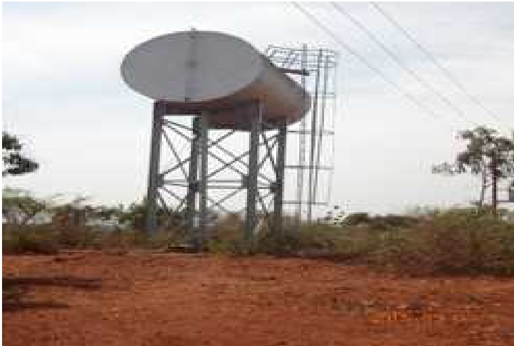
Plate 9: Reservoir 1 at Majanji Parish, Majanji Sub County.
