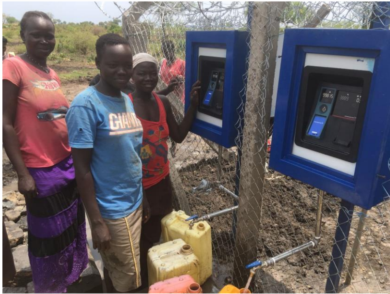
Photo: AQ Tap Installation in Bidi Bidi, Yumbe
