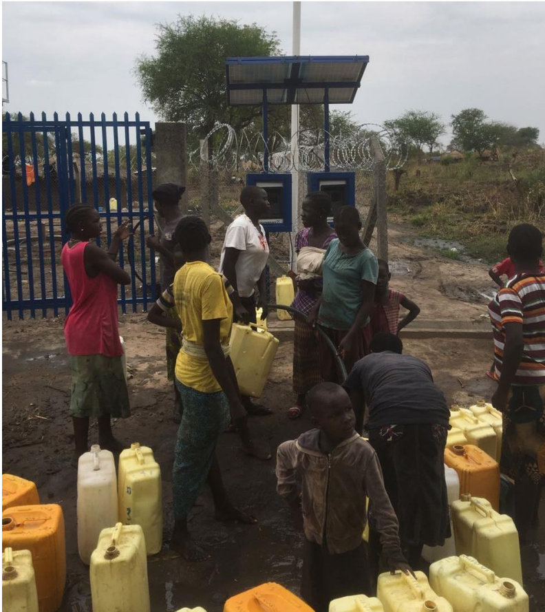
Photo: A scenario before commissioning of the system
