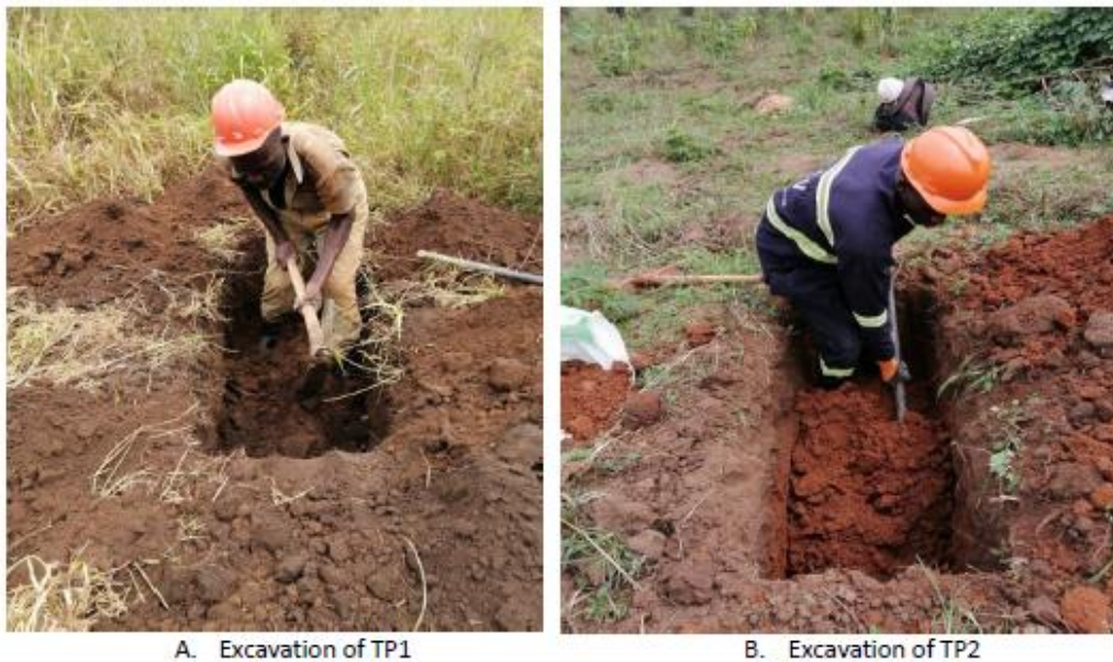
Figure 5: Excavation of trial pits
