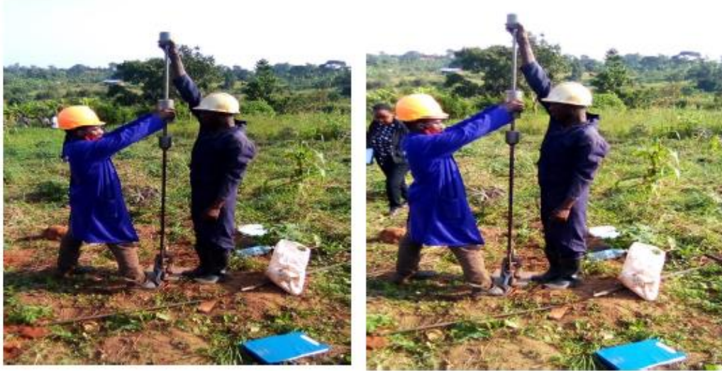
Figure 6: Conducting of the DPL test at site
