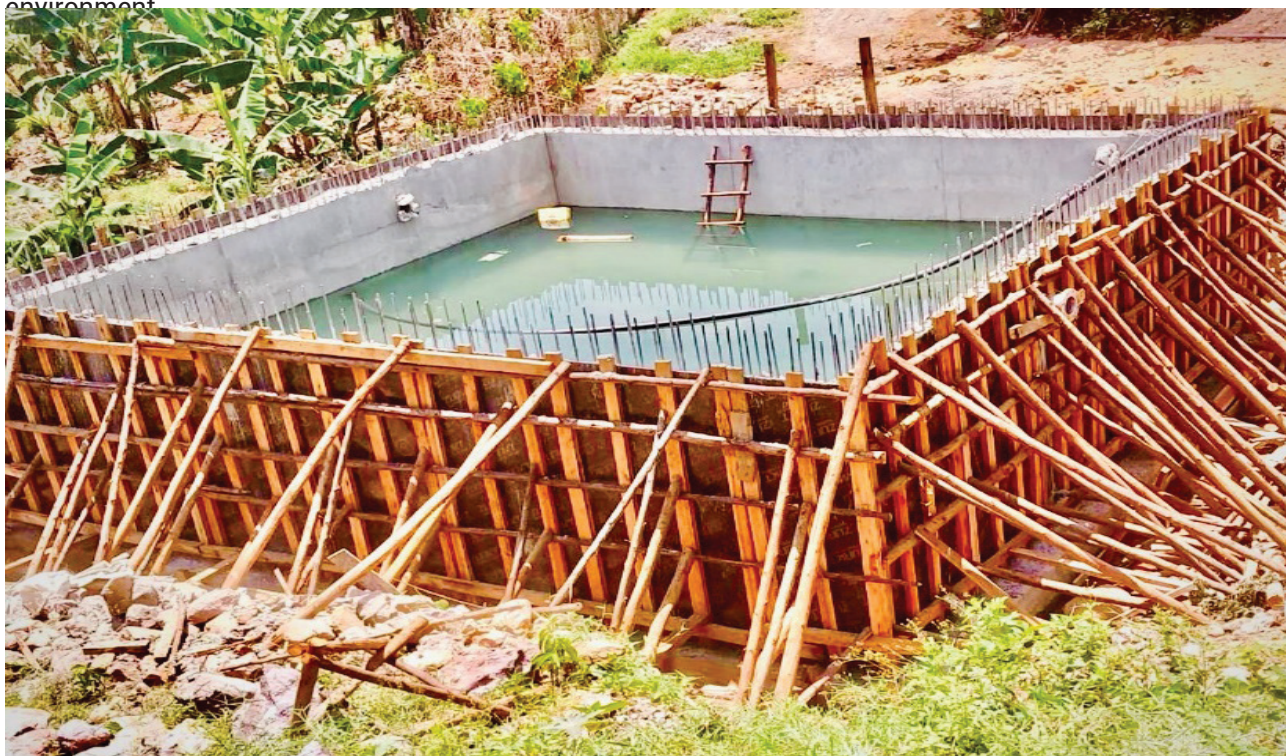
The new collection tank for Lunya Water Supply System under construction
