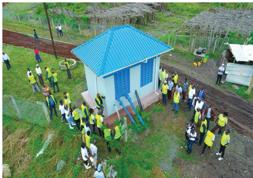
WSDF-Central staff together with Kagadi stakeholders inspecting the wash out at the pump house for Kagadi Piped Water Supply System
