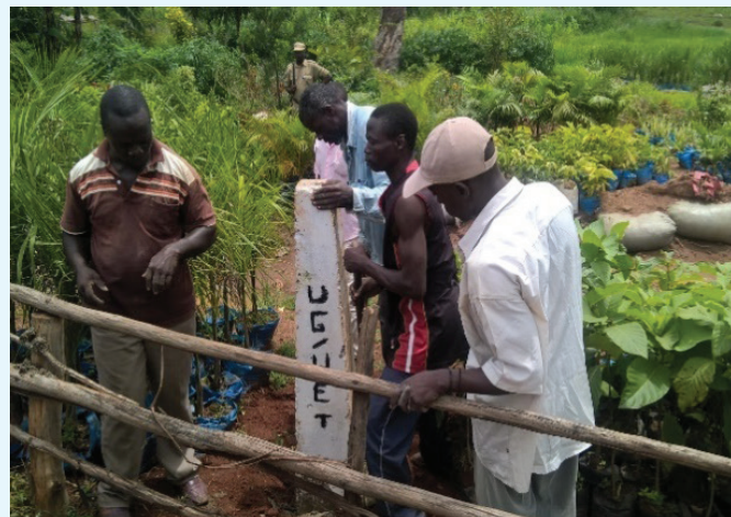
A pillar being installed in Mayanja-Kato Wetland boundary Restoration
