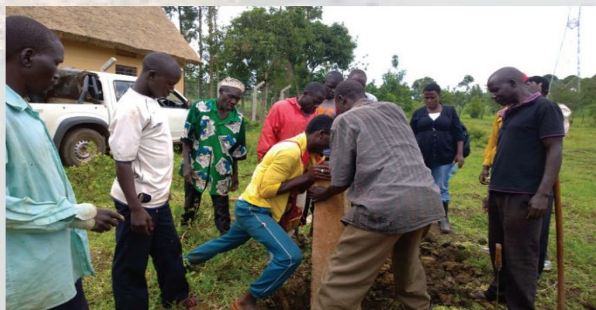
Pillars being lifted and planted.
