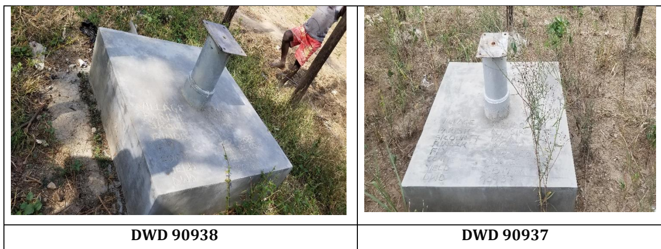
Plate 7: Drilled Boreholes in the project area
