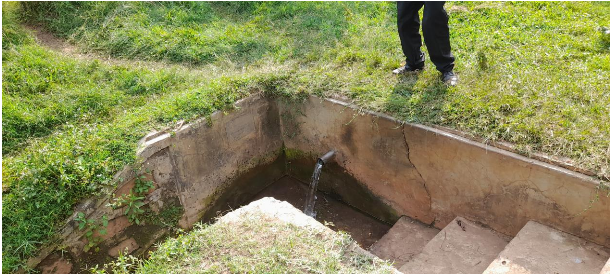
Plate 17: Protected springs in the project area, and Improvised spring “protection” as taken on 9 th February in Kyikyenkye
