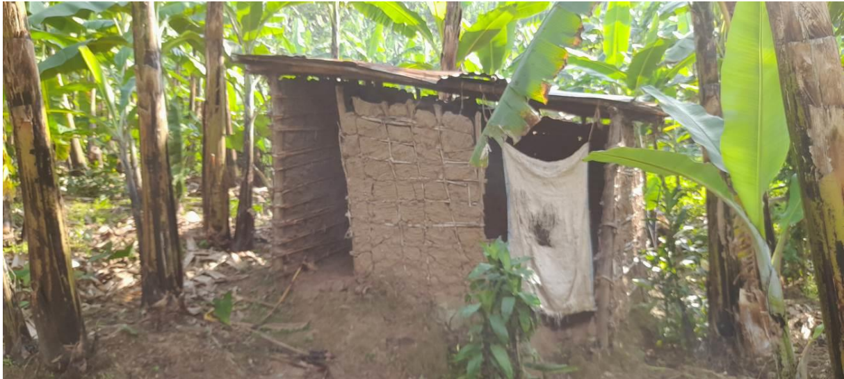
Plate 15: Poor latrine facility within the project area of Nyabuhikye
