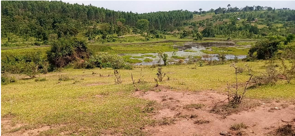
Plate 1: A view of the Kasensero Valley Dam
