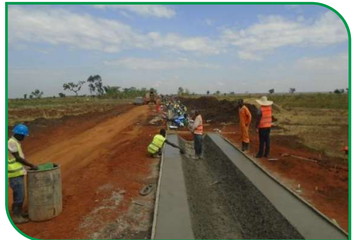
Concrete casting for secondary canal at Ngenge irrigation scheme, Kween district ■
