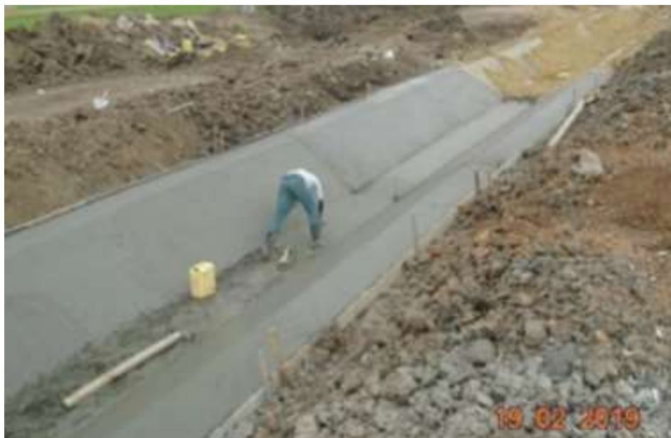
Concrete casting of canals at Doho II irrigation scheme, Butaleja District■
