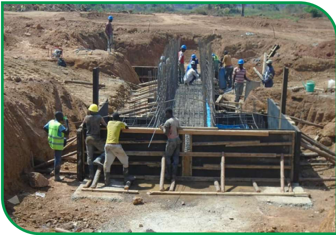
Construction of spillway at Tochi irrigation scheme, Oyam district ■
