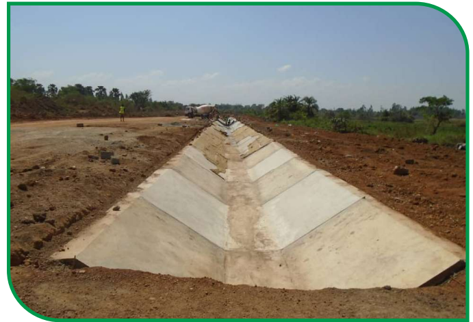
Concrete lining of main canal, Tochi irrigation scheme, Oyam district ■
