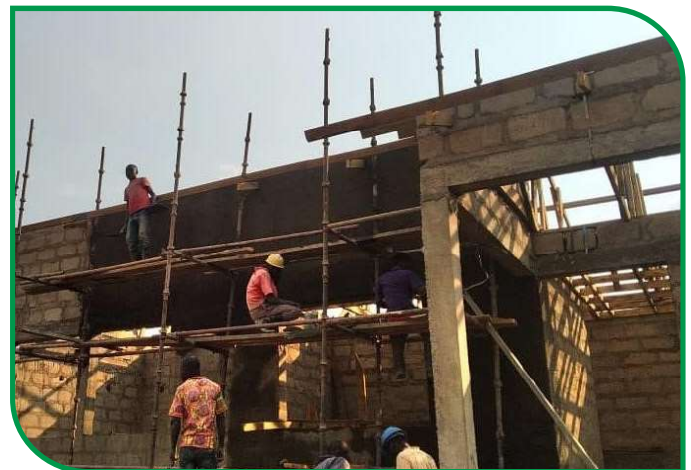
Ongoing construction of building at Wadelai irrigation scheme, Pakwach district ■
