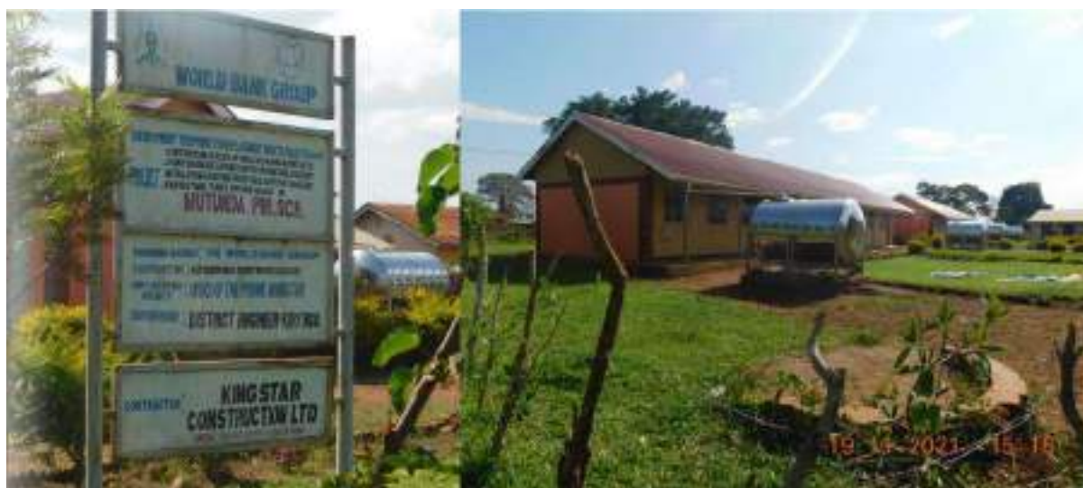
Figure 0-70: Steel water tanks at Mutunda primary School
