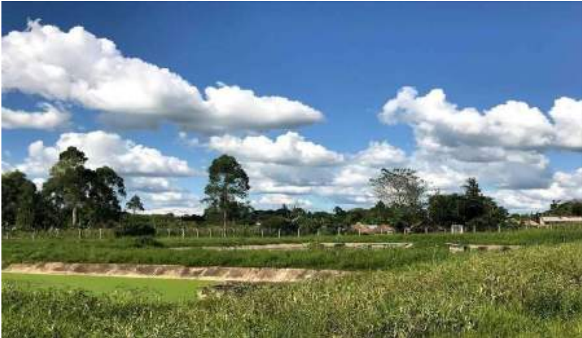
Figure 0-3: Waste Stabilization Ponds at Kiryandongo Hospital
