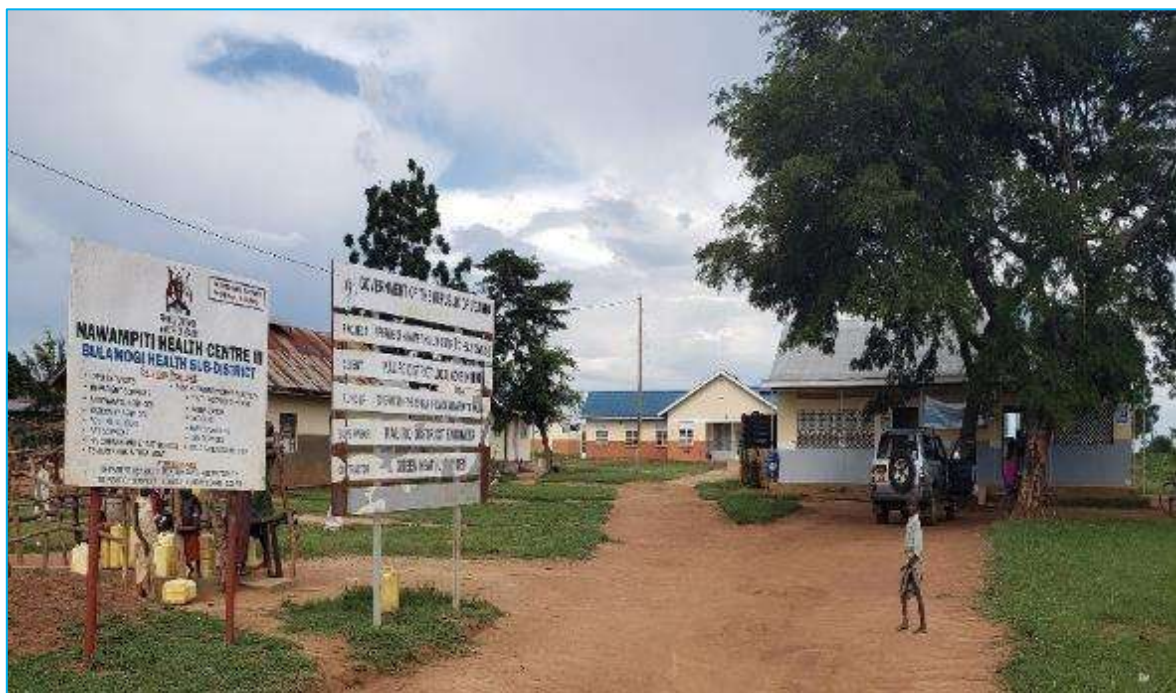
Figure 6-60: Nawampiti HC III in Bukamba Sub County
