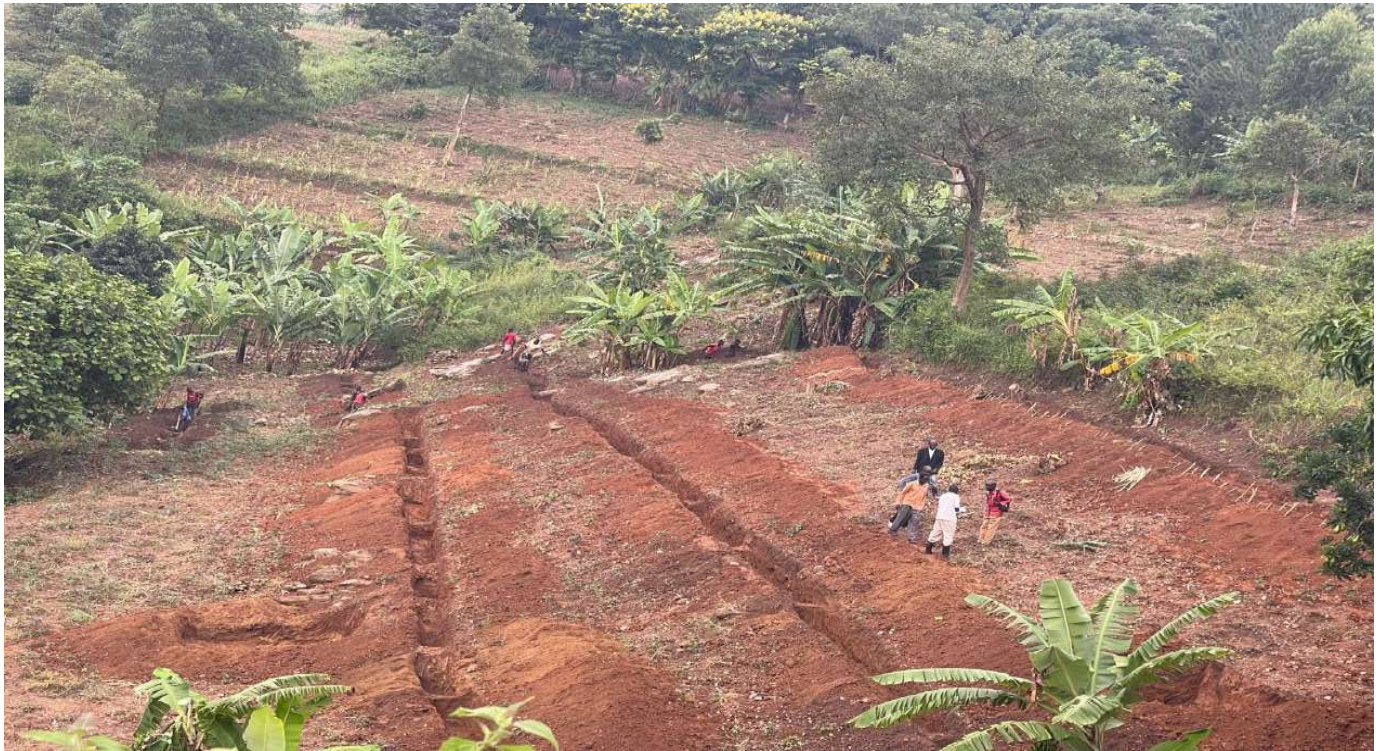
Demo sites for Soil and Water Conservation Structures in Erussi Sub-county, Nebbi District
