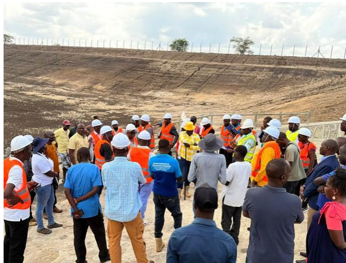
The delegation inspecting the completed spillway structure, embankments, and dead fence at Naitakiru Valley Tank.
