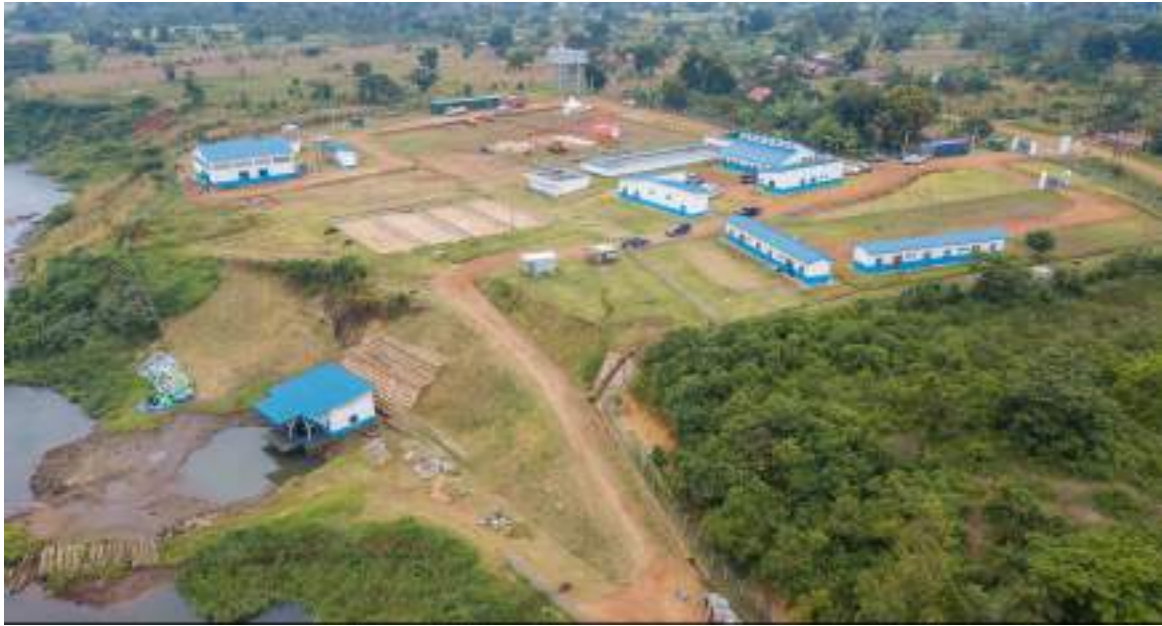
Aerial view of completed works for Kayunga-Busaana (Phase 1) Water Supply and Sanitation System, Kayunga district.
