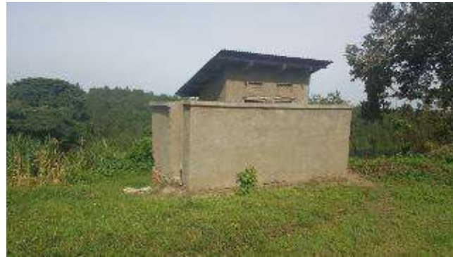
Latrine in Kihhi Town Council
