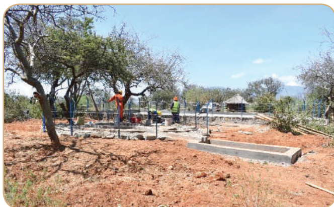
Compound water harvesting structures in Tapac f Moroto
