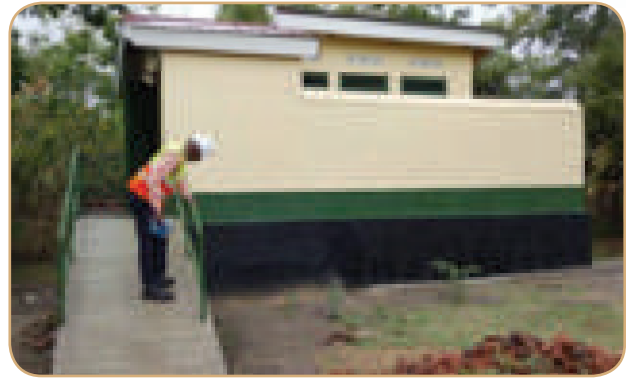
A newly Constructed latrine in one of the project schools
