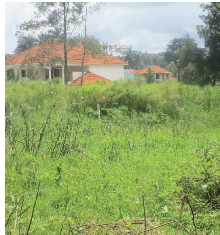
Plate 10: Building constructed in wetland
