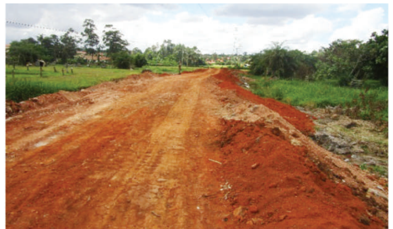
Plate 18: Dumping of murrum to create roads
