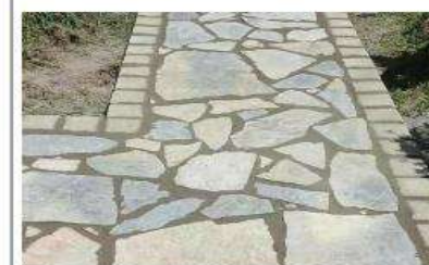
Examples of large natural stones in mortar
