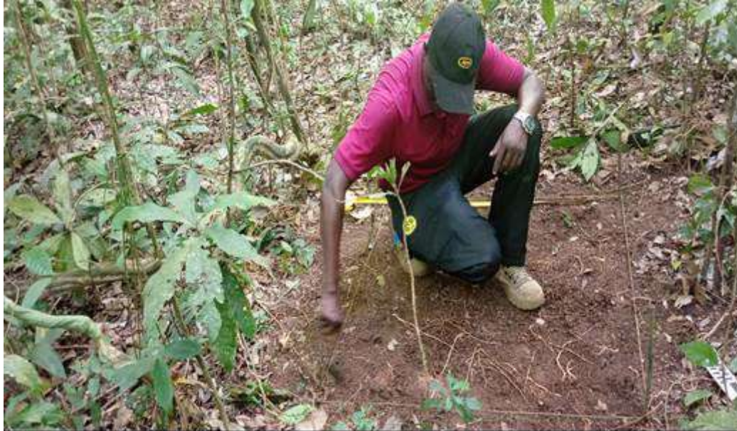
Figure 4-6: Test Pit Excavation in Progress
