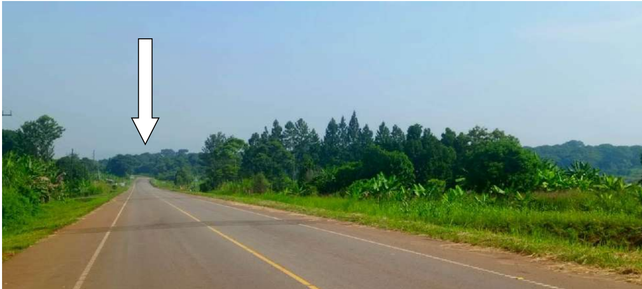
Figure 4-15: Approach Road to Kichumbanyobo gate
