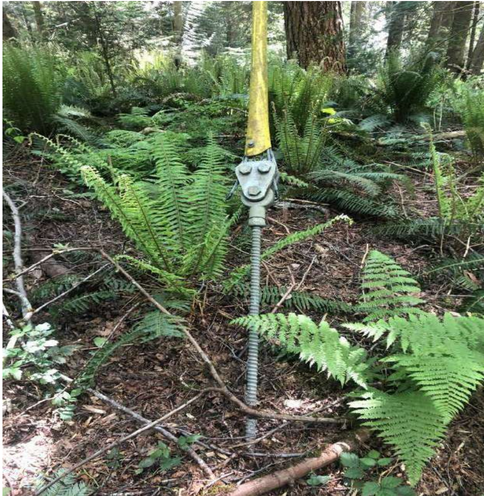
Figure 2-6: Micro pile anchor for canopy walkway
