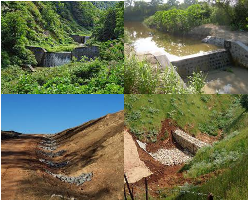
Figure 5 - Sample of Check Dams
