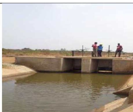
Photo 7.2-2: Installation of sluice gate at cross regulator 1 at Wadelai Irrigation scheme in Pakwach District
