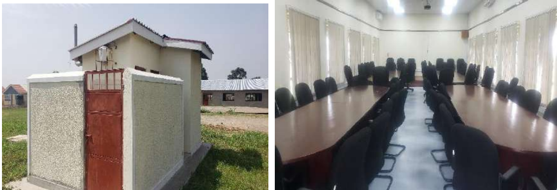
Photo 3-5: Completed Toilet block and Conference Hall
