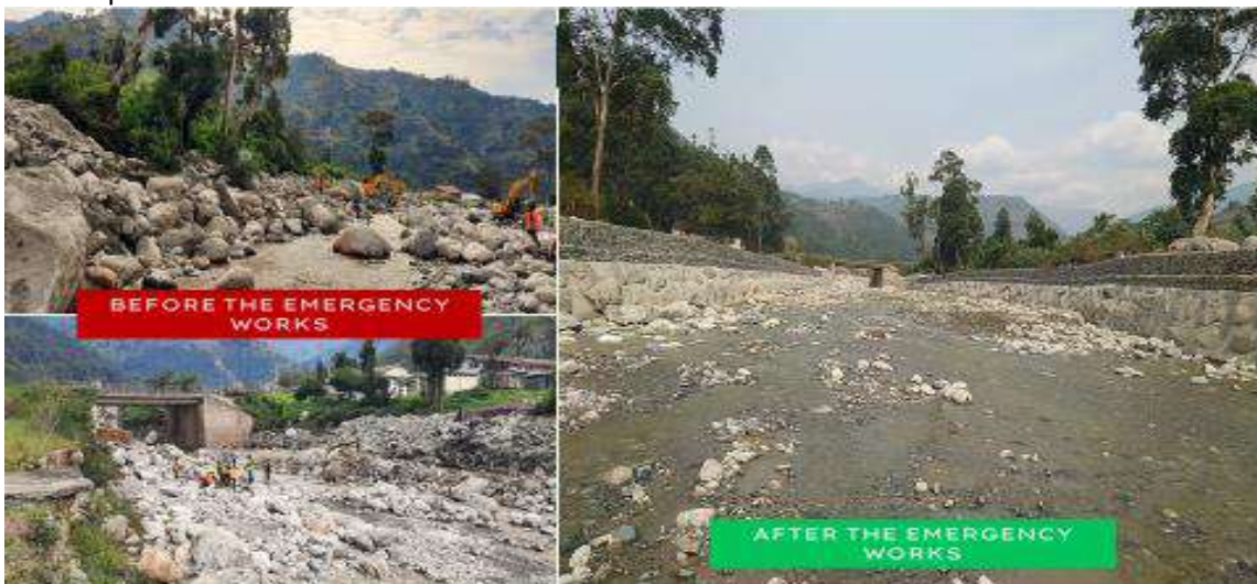
Photo 3-8: Emergency maintenance works for R. Nyamwamba
