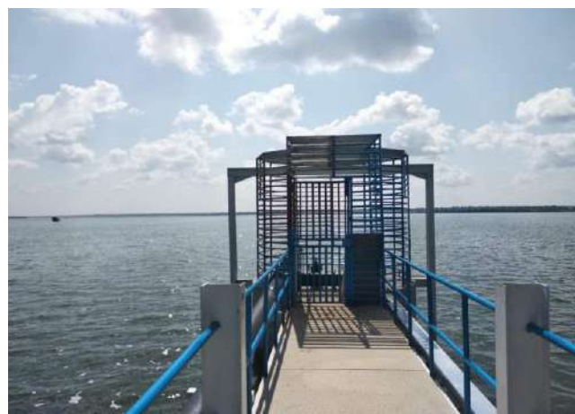
Picture 4.2: Completed structure with security cage installed
