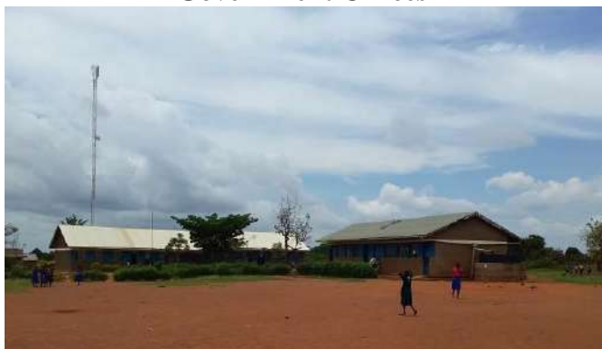
Picture 2.12: Banda Sub-county Offices
