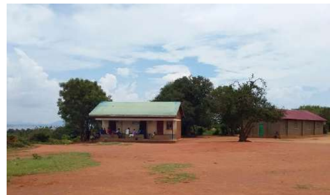
Picture 2.13: Banda Sub-county Offices
