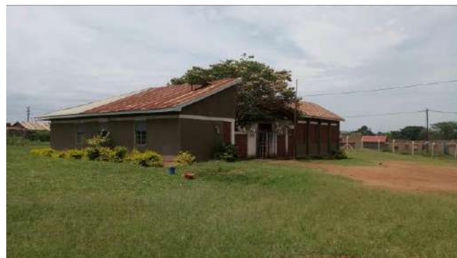
Picture 2.11: Banda Sub-county Offices
