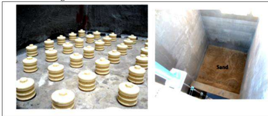
Figure 4.4: Filter Nozzles and Sand Bed
