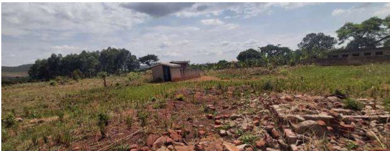
Figure 5-16: VIP pit latrines at Bugomolwa Primary School.
