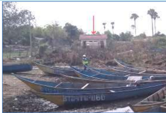
Damaged public toilet at Iyingo Landing site
