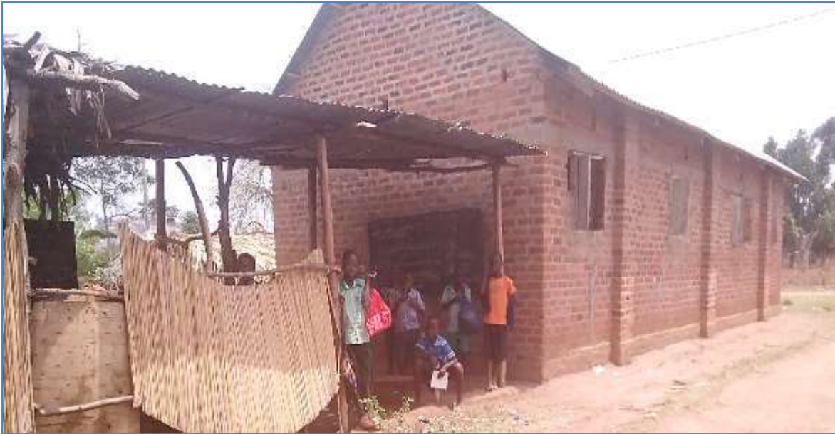
Figure 6-67: Buyumba Nursery School faces severe water scarcity
