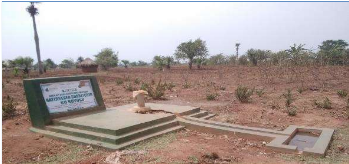
Figure 6-54: Non-functioning deep borehole at Bumogoli village
