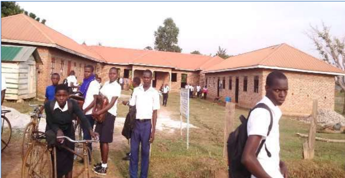
Figure 6-68: A secondary school (Kagulu Hills College) with no RWHT in Igwaya RGC
