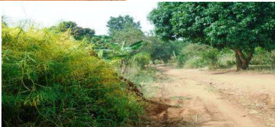
Landscape cover along the Transmission corridor through Mailo
