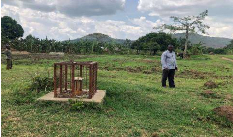
Figure 5-17: Nakasero production well in Bananywa Subcounty.
