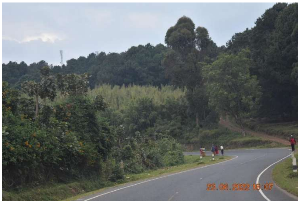
Plate 4.3: Access to the project site off Kabale – Kisoro Road
