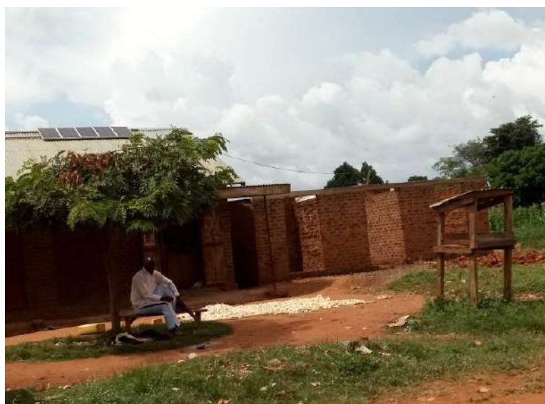
Picture 2.7: Solar Panels on house top in the RGC
