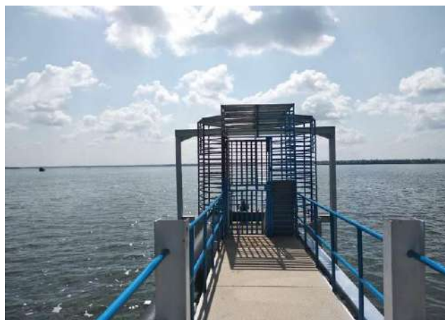
Picture 4.2: Completed structure with security cage installed
