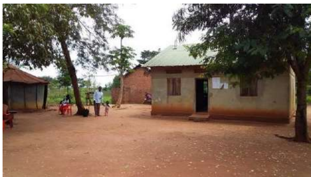
Picture 2.12: Bukamba Sub-county Offices
