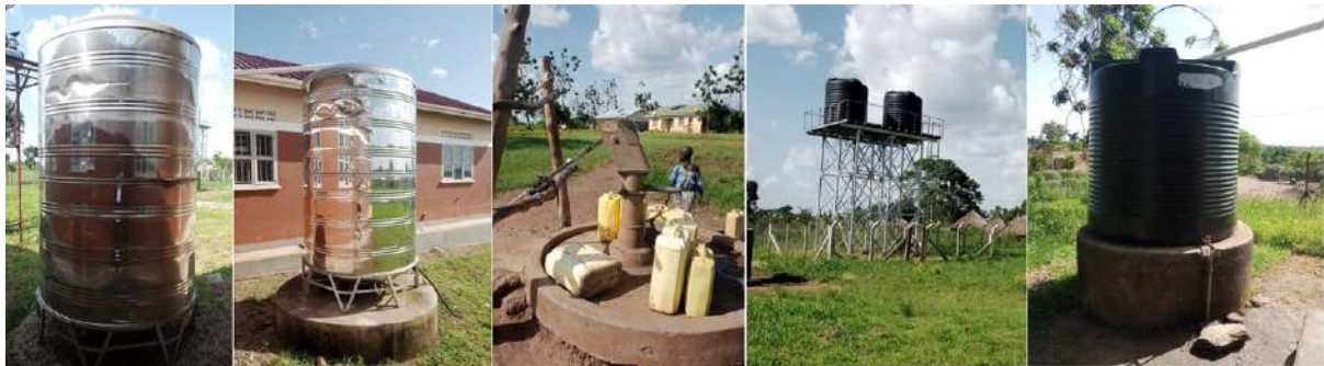
Figure 5-69: RWHTs, Borehole, Storage tanks at Apodorwa HC III with support from OPM/DRDIP/ World Bank
