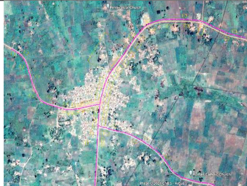
Aerial view of Apodorwa area
