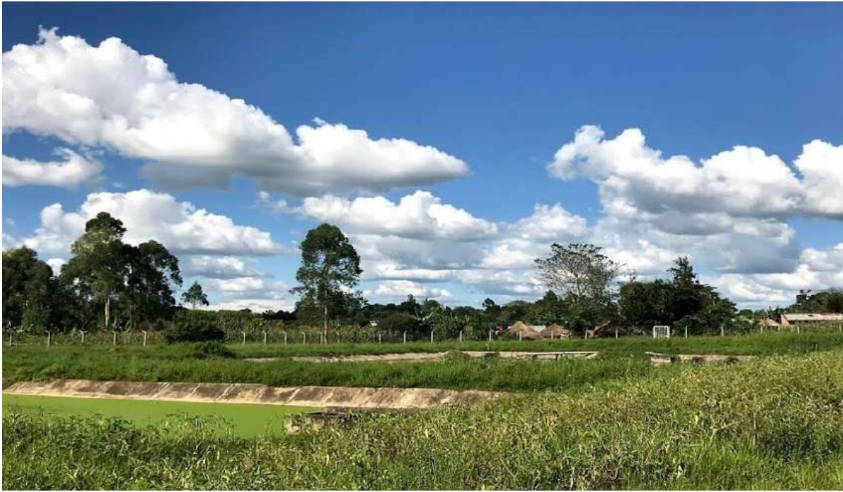
Figure 7-3: Waste Stabilization Ponds at Kiryandongo Hospital
