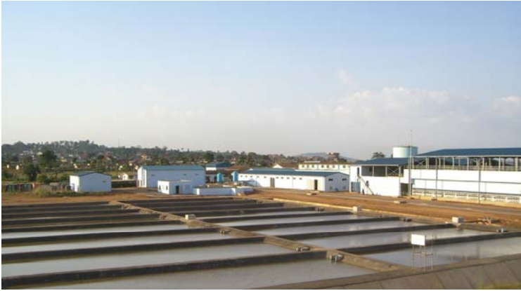
NWSC's new Gaba III water treatment plant
