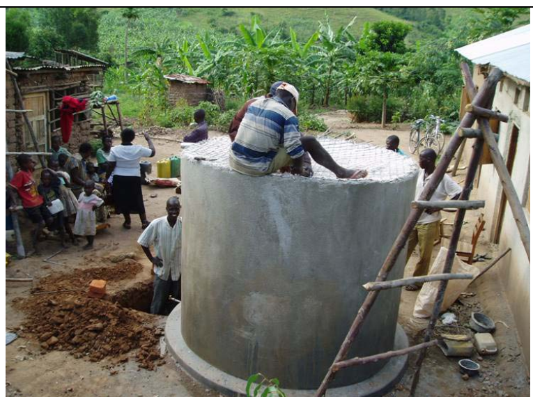
Family RWH tank being completed – without walking distance to access it
