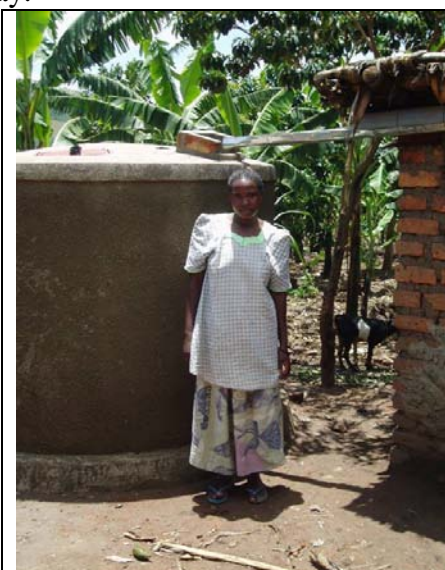
Completed tank within no walking distance
